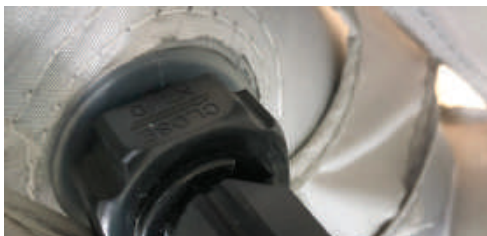
To OPEN valve turn counter clockwise. To CLOSE valve turn clockwise until firm.
