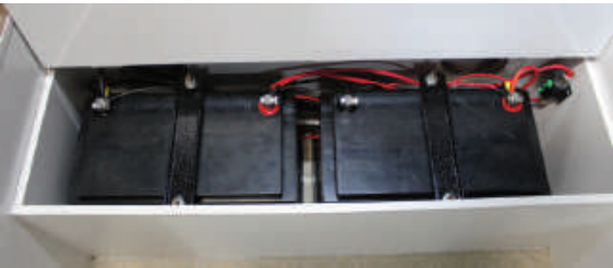
Batteries 2x 100Ah deep cycle AGM batteries with 240V charger
