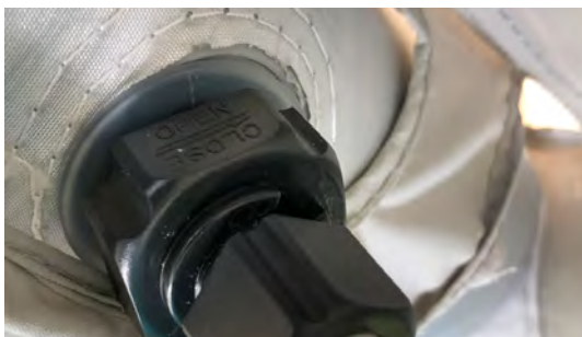
To OPEN valve turn counter clockwise. To CLOSE valve turn clockwise until firm.
